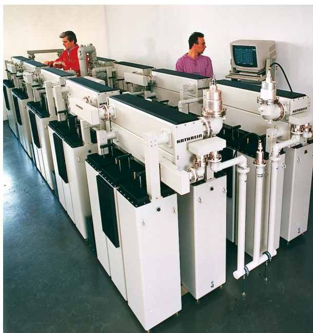
Combiners and layout for Marlow transmitter in Germany. Multi-pattern antenna system for 7 FM channels.
