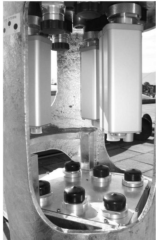
View inside service zone with MPTMA and Slimline RCUs
